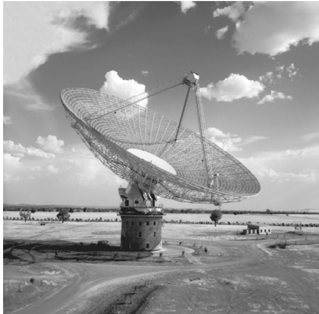
Figure 9: The Parkes Radio Telescope, completed in 1961, supported the Mariner 2 mission to Venus in 1962. Its design was the prototype for the DSN's 64-m tracking antennae. Credit: CSIRO/ATNF
